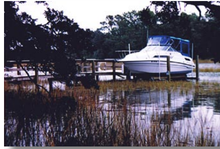
8000 LB. ELECTRIC BOAT LIFT ALONG SIDE THE 90' PIER
